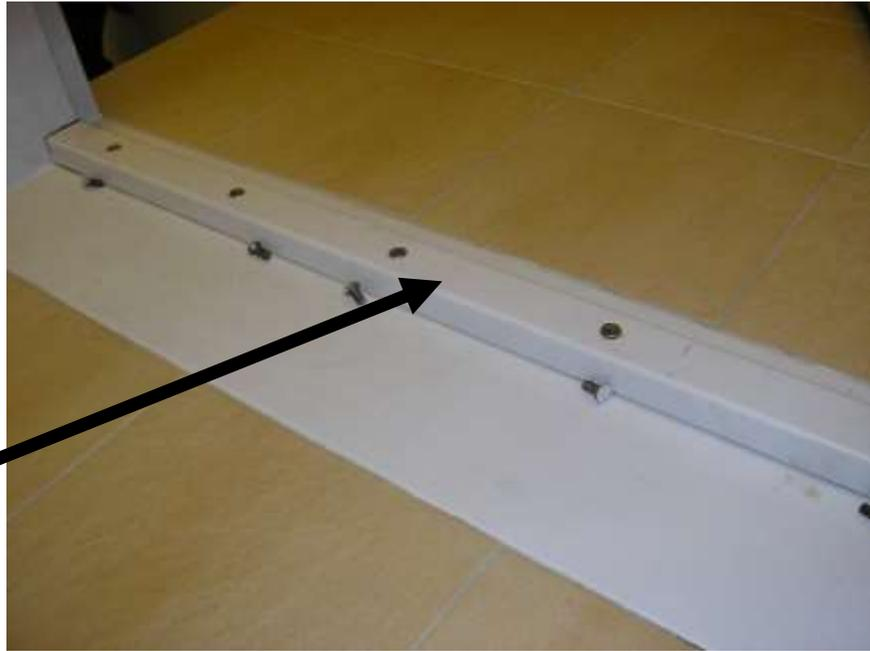
Install door kerb on bottom edge of SS door.
