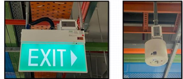
Sensor for Emergency Light / Exit Sign
