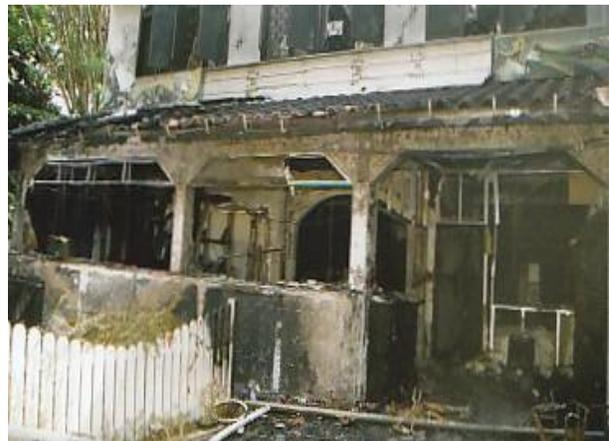
**Figure 17.** Other parts of the building sustained heat, smoke and water damage
