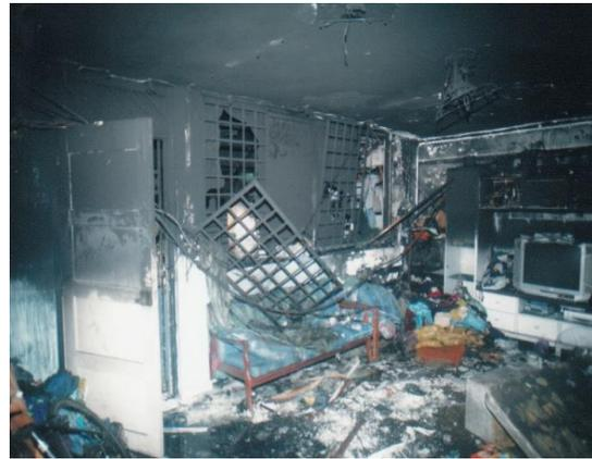
**Figure 9. Other parts of the unit sustained severe heat and smoke damage**
