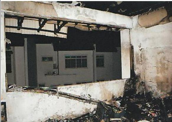
**Figure 14. Fire damage was severe in the master bedroom**
