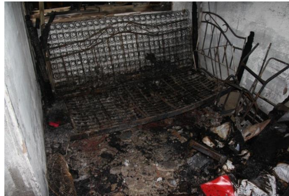
Figure 21. Burnt remains of the powerbank were recovered in the Area of Fire Origin
