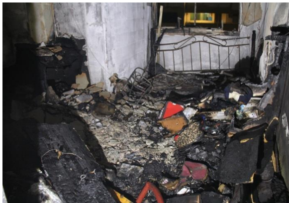
Figure 18. The contents of the room were damaged
