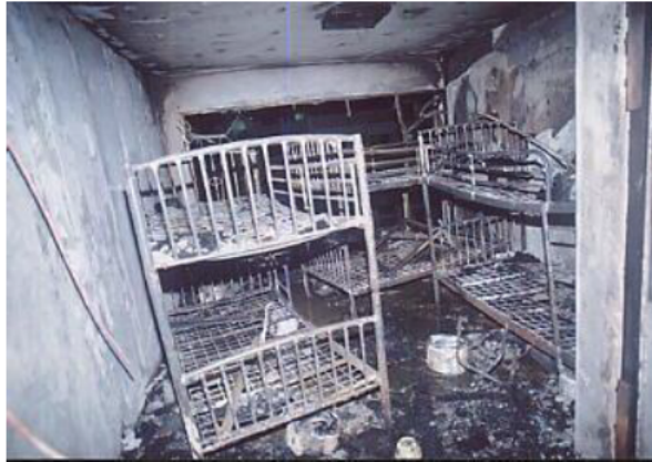
Figure 10. A section of the living room was partitioned up and used as a bedroom
