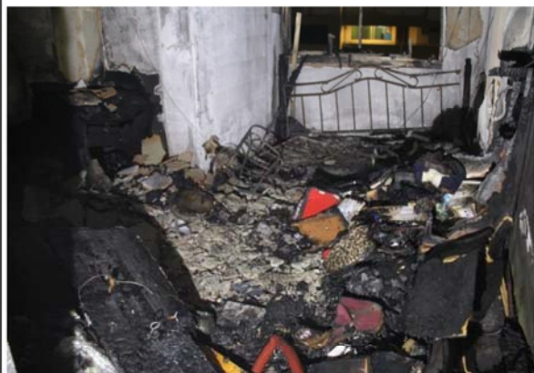
Figure 18. The contents of the room were damaged
