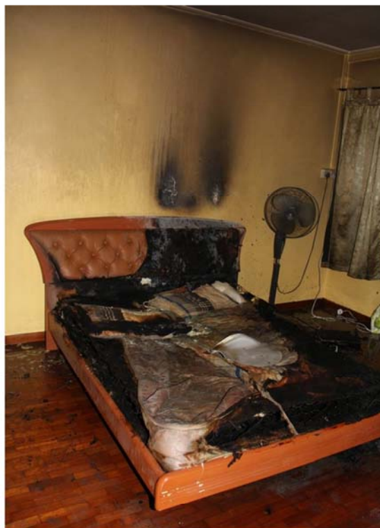
Figure 22. As a result of the fire, the bed was damaged. The walls and flooring in the room sustained heat and smoke damage
