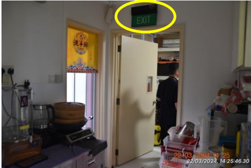
Exit Light not in proper working order
