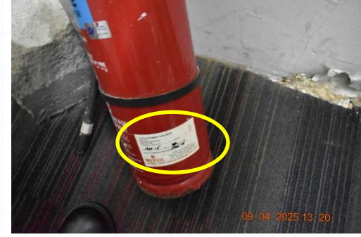
Fire Extinguisher not serviced
