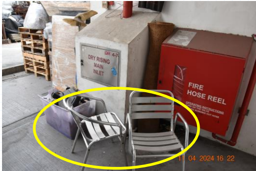
Obstruction to breaching inlet and hosereel
