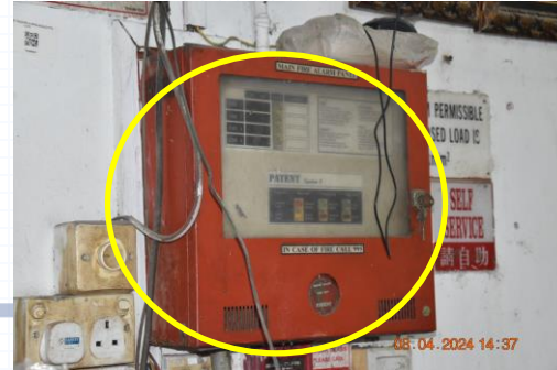
Fire Alarm Panel not in proper working order
