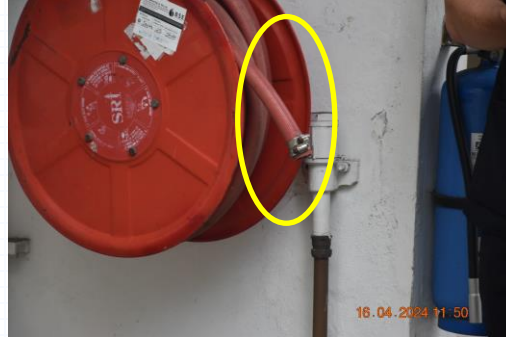
Hosereel nozzle missing
