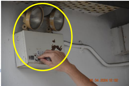
Emergency Light not in proper working order
