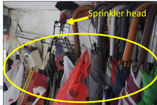
Obstruction to sprinklers head
