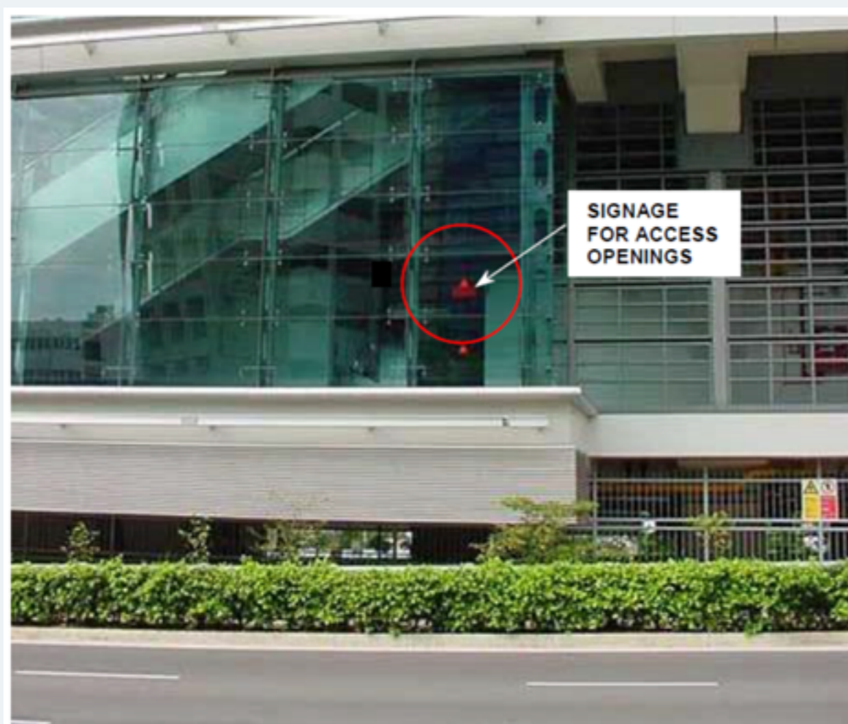
The access openings signage provided on the external side, either red or orange triangle would help firefighters on the ground to locate the designated access openings.
