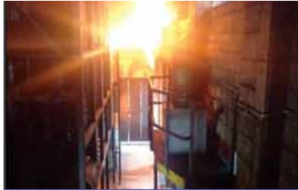
High Bay Storage (Level 4)
