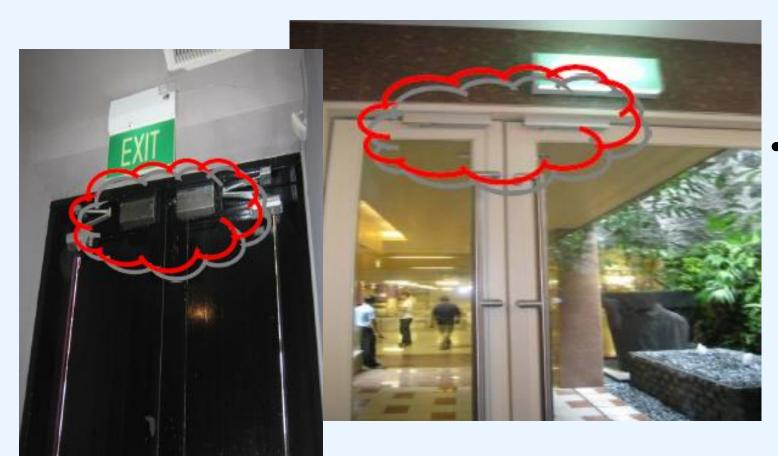
Under alarm activation mode, the electro-magnetic locks are not activated to unlock the exit door
