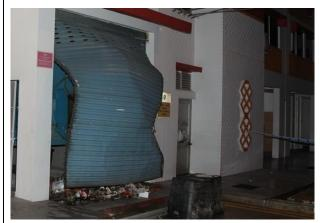
Figure 12. The roller shutter of the bin centre was observed to have bulged out
