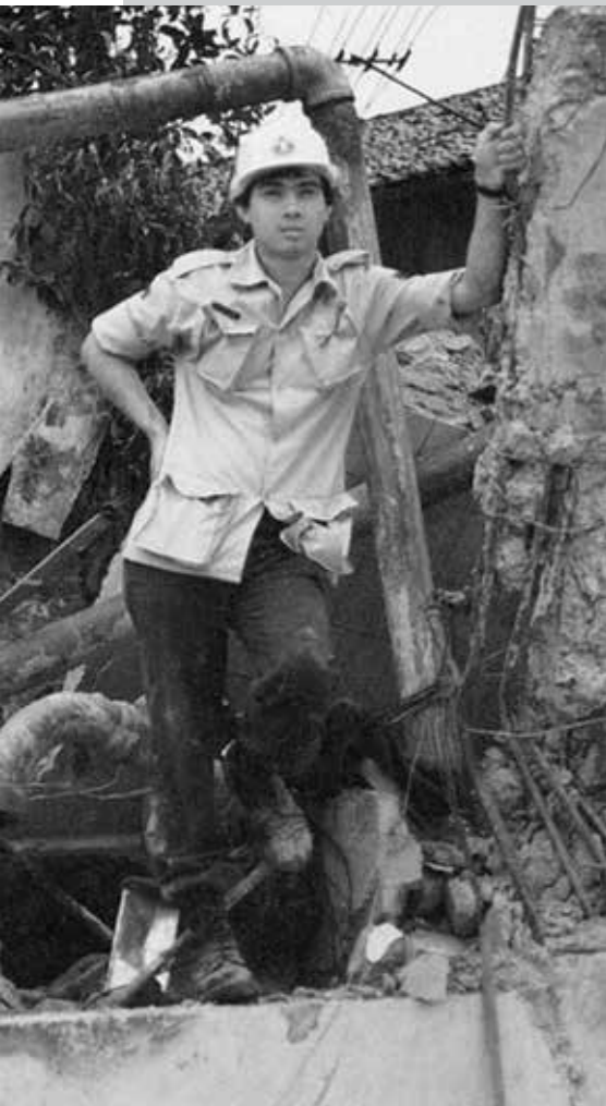
Mr Tan Kim Teck at the Hotel New World collapse incident site.
